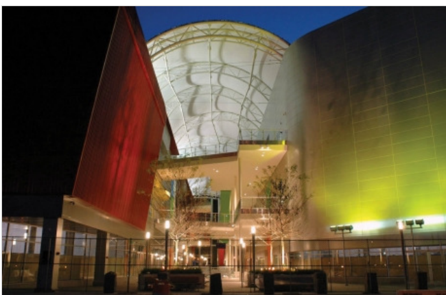
Truss arches span two different types of building systems over a pedestrian walkway at Vornado's Rego Park Retail Center atrium
