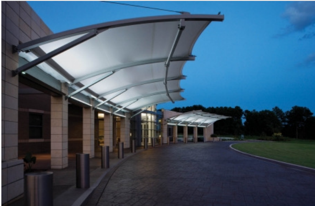
A custom cantilever canopy attached to a main structural system shades a drop-off area at the Magnolia Medical Plaza in Palestine, Texas. Architects: WHR Architects; Fabricator: FabriTec Structures.
