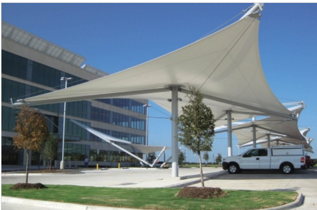
Custom structures with high-end paint finished steel and vinyl-coated polyester hypars shade Valliance Bank's entry and carpark in Dallas, Texas. Architect: TAP Architects; Fabricator: FabriTec Structures.
